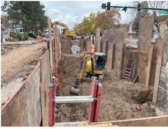
Work area showing the opening where the tool was inserted into the pipeline.
